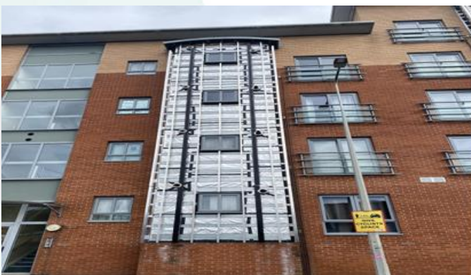
B2 Now Ready For Fire Stop & Insulation
